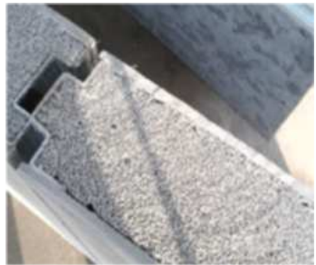
Panel cross-section view
