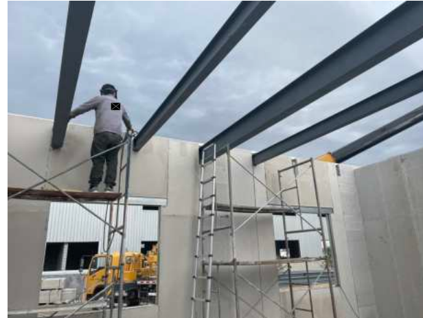
Wall panels with sealed joints and factory pre-fabricated steel A-frames, purlins and beams
